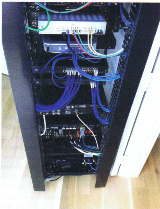
The original wireless network was insufficient, so Eco High Fidelity in Richardson, Texas, used Pakedge equipment to create VLANs to support Crestron and Kaleidescape.
